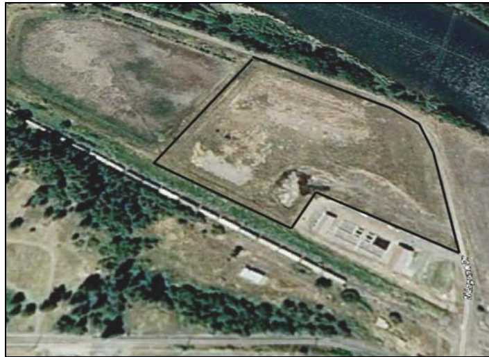
City Site #2 (between RR track and river)
